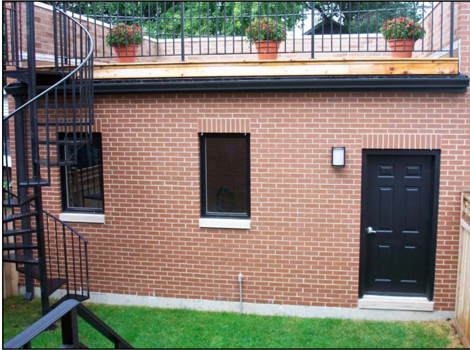
Yard & Deck Over The Garage
